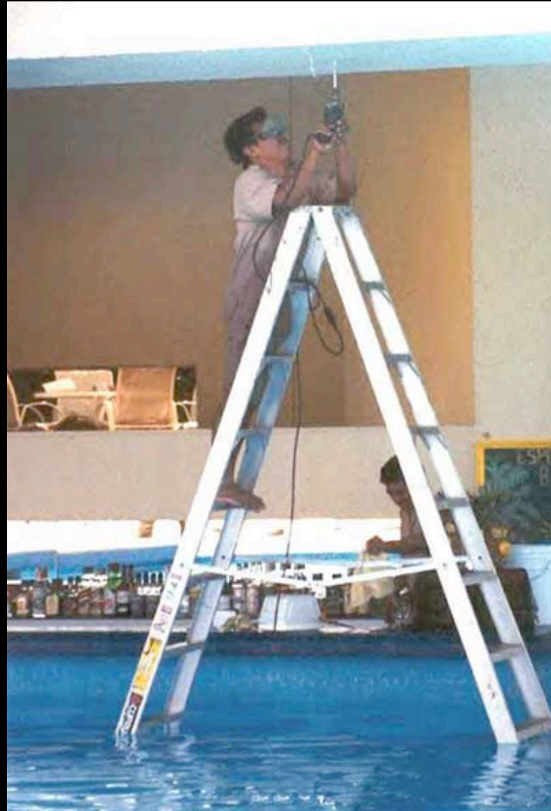
Moron: Using an electric tool, in a pool, with a metal ladder. Stupid Moron: Standing barefoot on the ladder while doing it.
